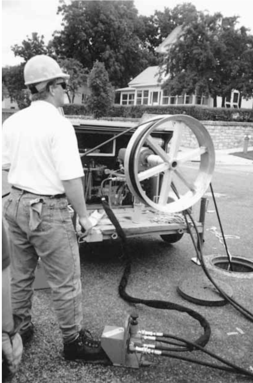
Figure 4-8 For long pulls, the mechanical puller applies consistent tension and monitors it to prevent overstressing the fiber.
